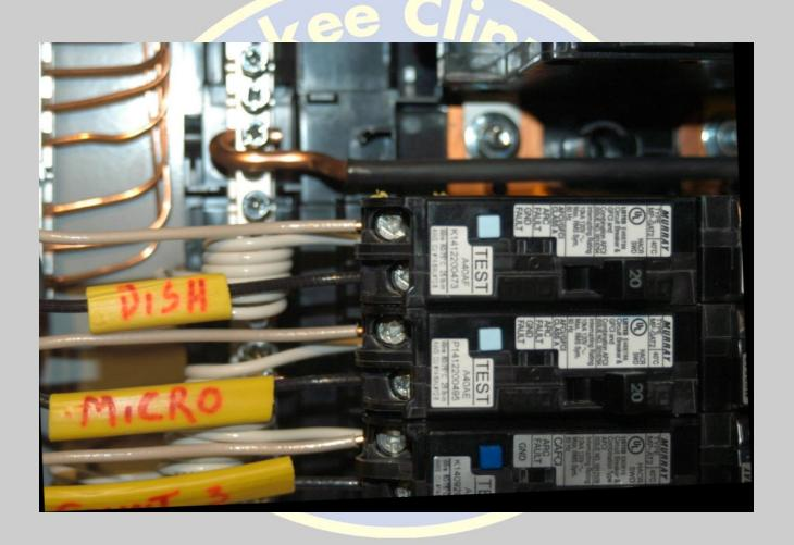
Four-terminal device, with Line Hot and Neutral, Load Hot and Neutral
